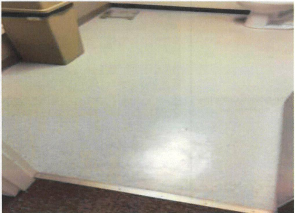
Non-Asbestos Vinyl Sheet Flooring in Main Floor Washroom
