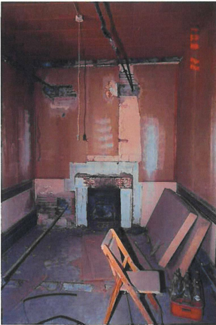
15. ROD "TENSION" TIES AT SECOND FLOOR LOOKING EAST TOWARDS CORRIDOR WALL.
