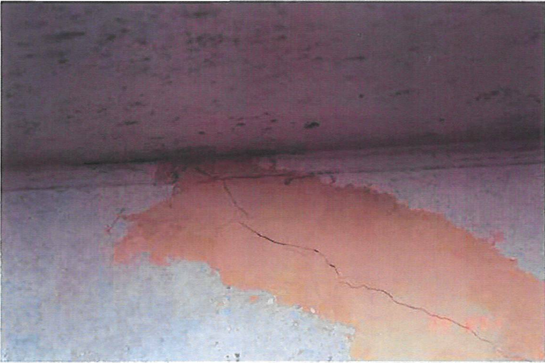
25. MAIN FLOOR BEAM IN VAULT BASEMENT UNDER PHOTO 23 - WEST FACE.
