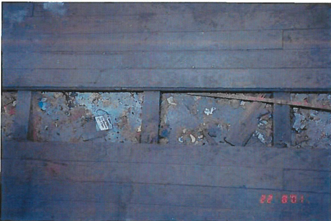
18. SECOND FLOOR BOARDS, SLEEPERS AND ASH FILL AS "ACOUSTIC" TREATMENT.
