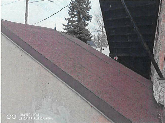
Figure 1 – Overview Roof A1
