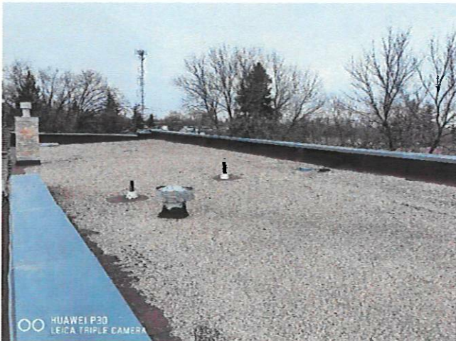
Figure 3 – Overview Roof B2
