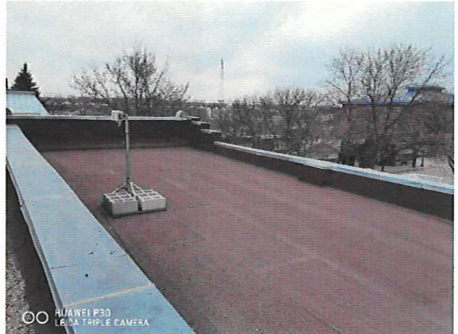
Figure 2 – Overview Roof B1
